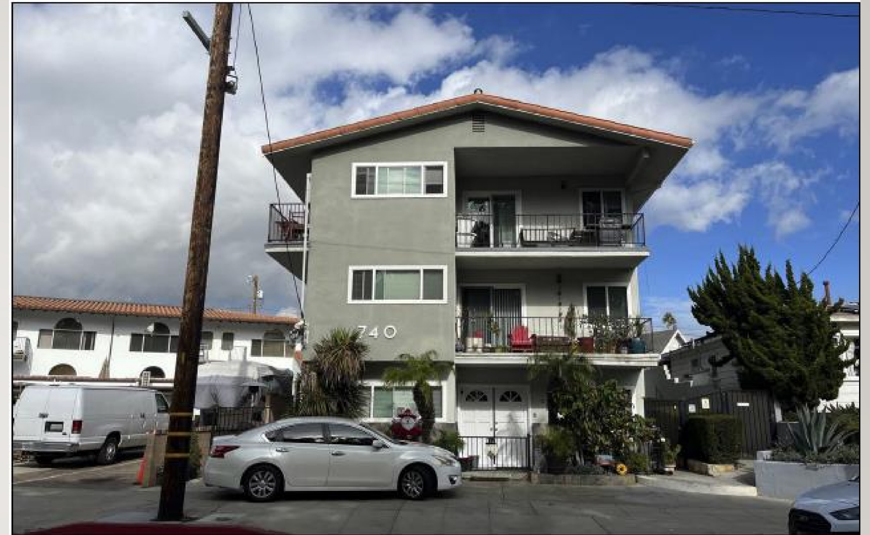
740 Paseo del Mar, built in 1962 – 33.7 feet tall*, 67.7% lot coverage
