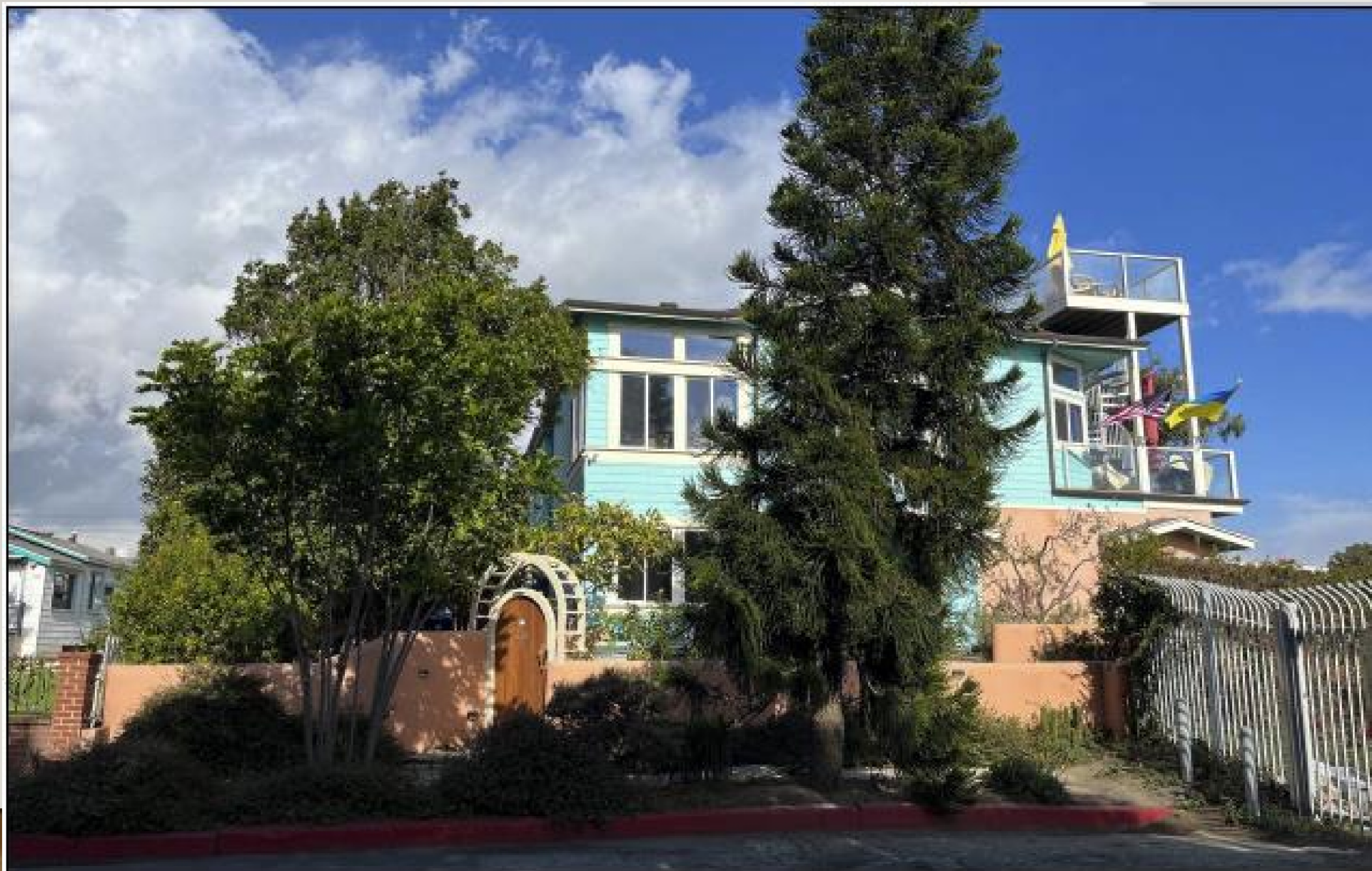
670 Paseo del Mar, built in 2005 – 26 feet tall, has roof deck and ADU, 32.3% lot coverage
