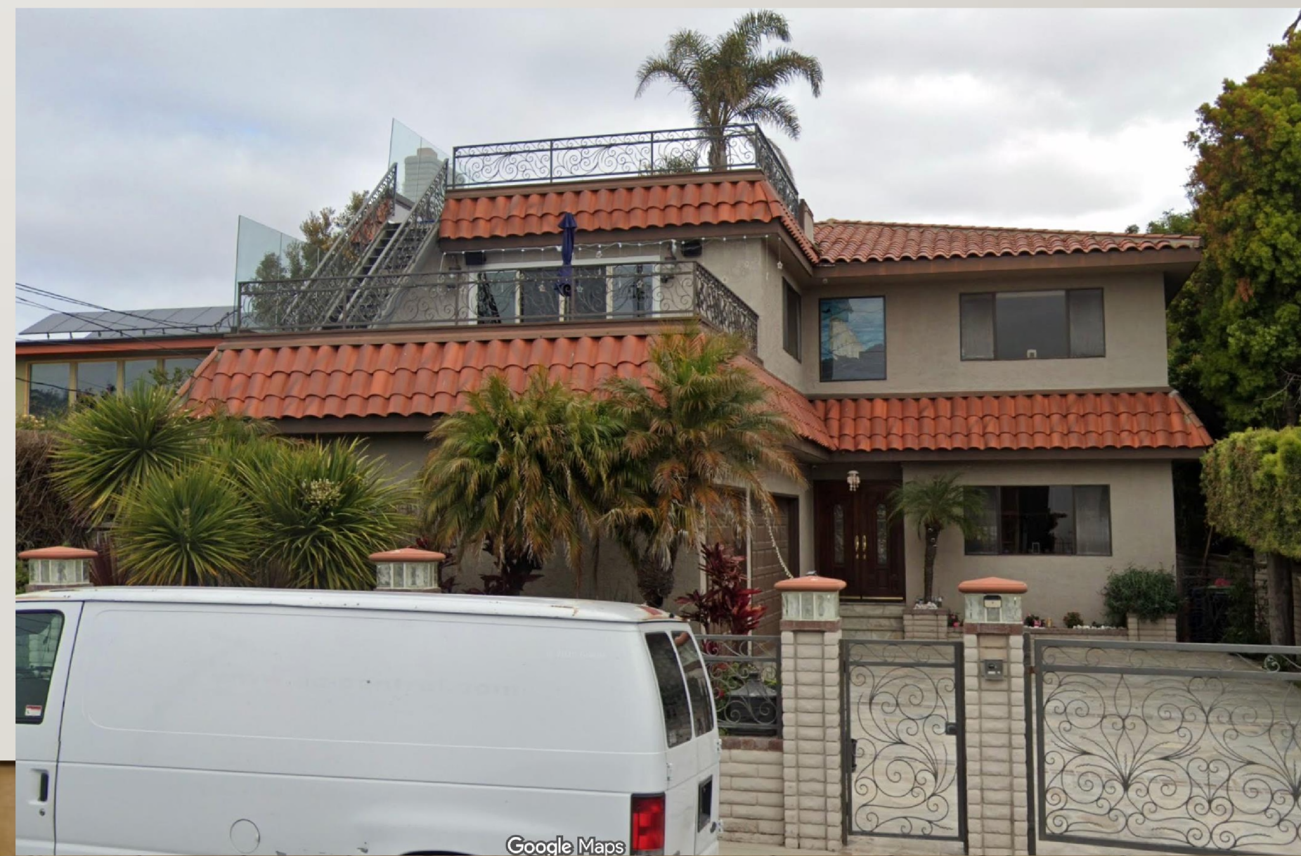
548 W Shepard St, built in 1979 – 28 feet tall, has roof deck
