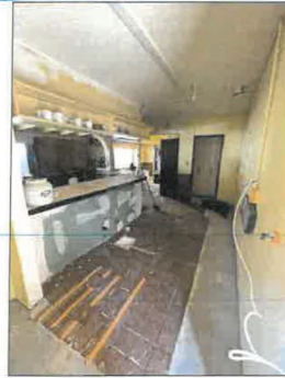
② EXISTING TILES TO BE REMOVED AND REPLACED
