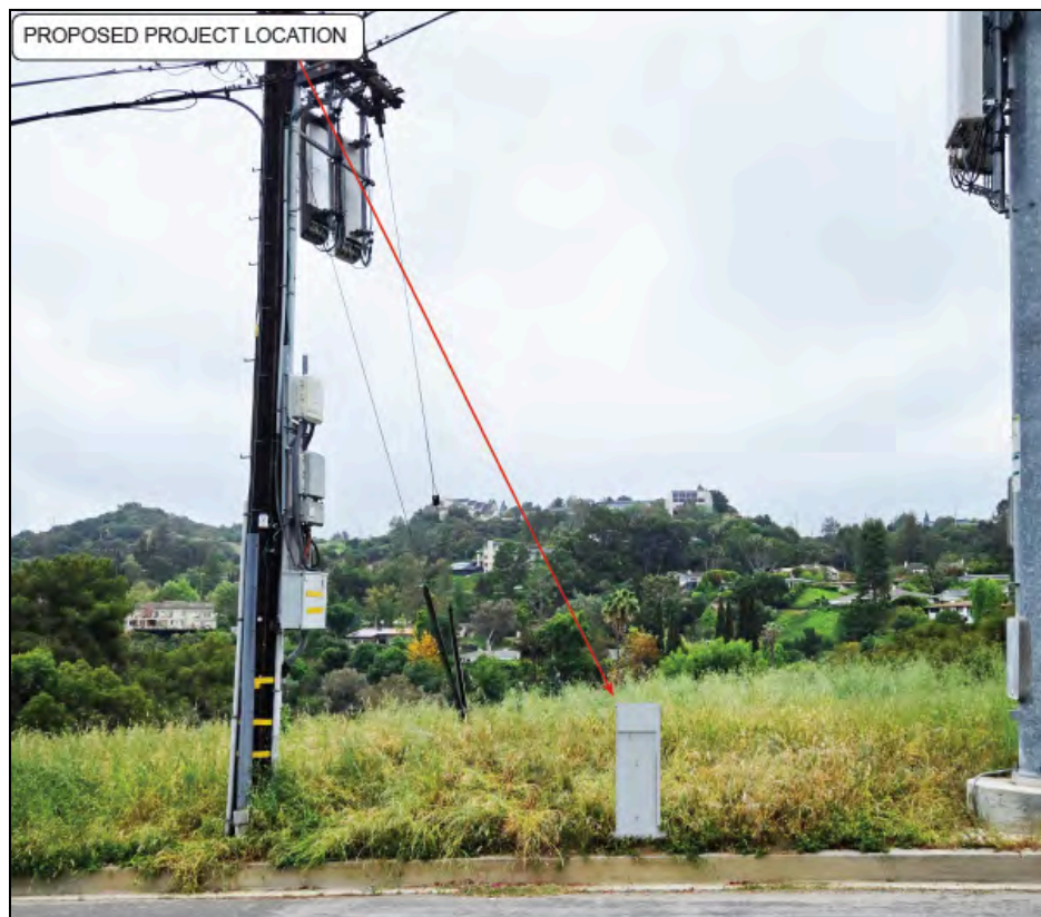
Figure 1. A red arrow points to a rendering of the proposed AGF Cabinet. The utility poles to the left and right are existing utility poles.
