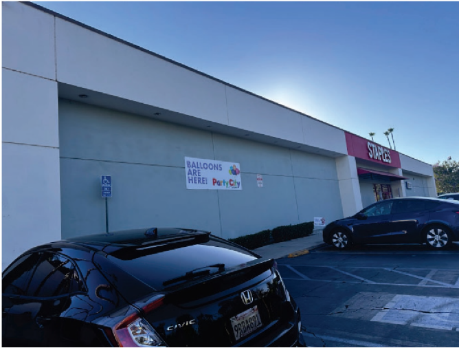
Representative view of the Staples building, which has relatively modern architecture lacking crevices and cavity spaces consistent with the buildings found throughout the rest of the project site.
