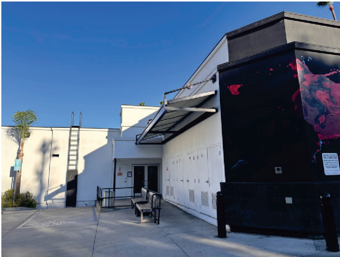
Representative view of the backside of the Pinz bowling and restaurant building, which has relatively modern architecture lacking crevices and cavity spaces consistent with the buildings found throughout the rest of the project site.
