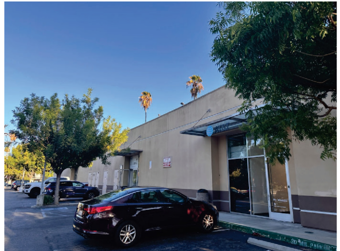
Representative view of the building at the eastern end of the site, which has relatively modern architecture lacking crevices and cavity spaces consistent with the buildings found throughout the rest of the project site.
