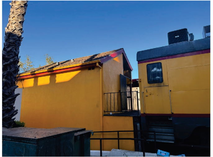
View of the roof shingles at Carney's Restaurant. Some of these roof shingles contain crevices that could be used by day-roosting bats; however, no bats emerged from these shingles during the nighttime survey.
