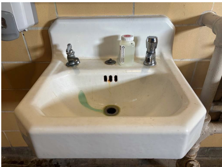
Lead in Water Testing Location - Pool House Women's Bathroom Left Sink
