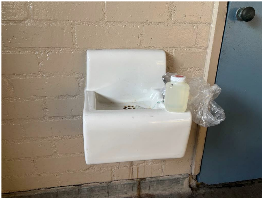
Lead in Water Testing Location - Pool House Men's Changing Area Drinking Fountain (30-Second Draw)
