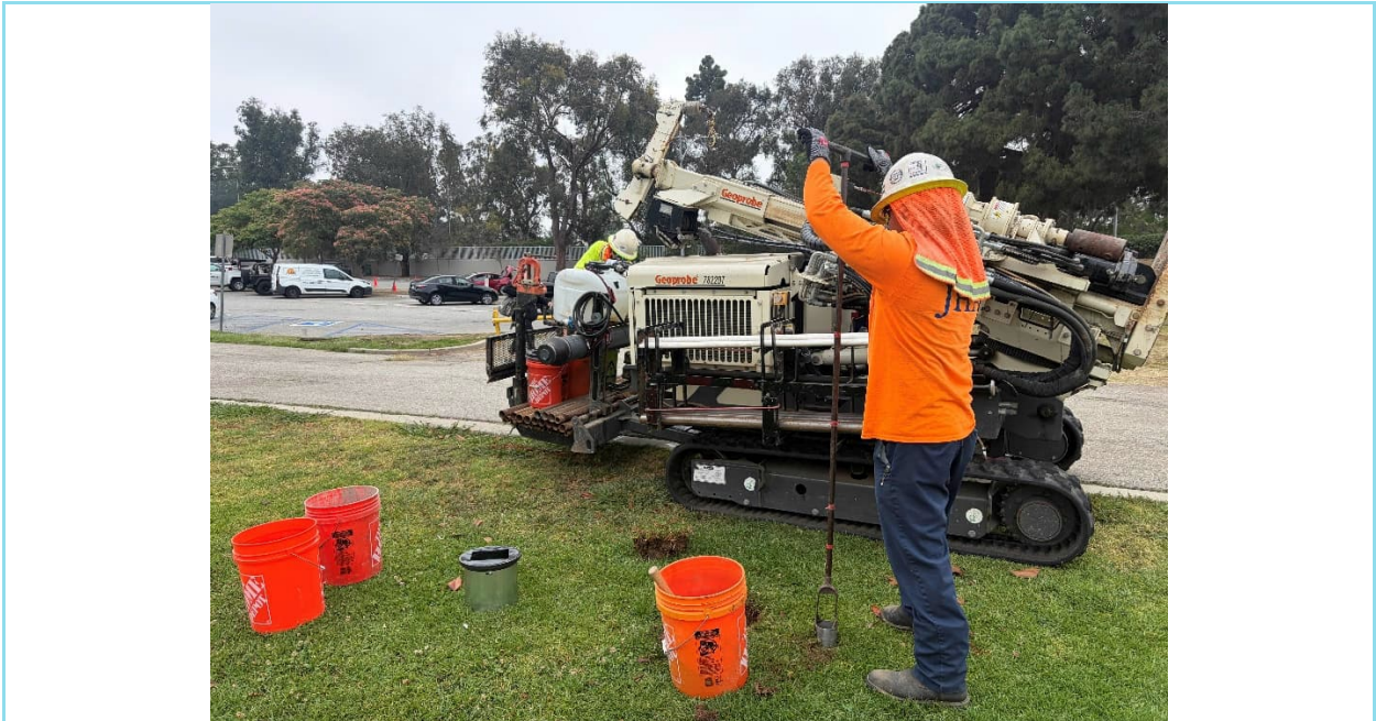
Photo 2: Drilling at SGP-1 and SGP-2.
