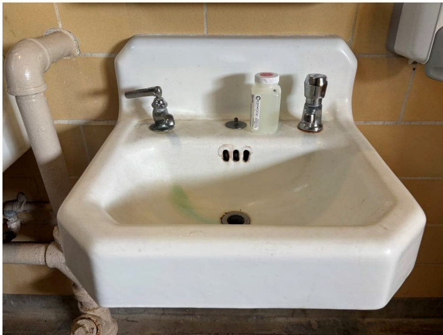
Lead in Water Testing Location - Pool House Women's Bathroom Right Sink
