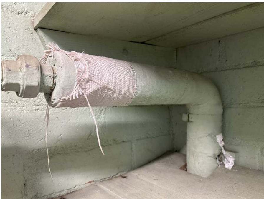
HA 2 - Water Pipe Insulation
