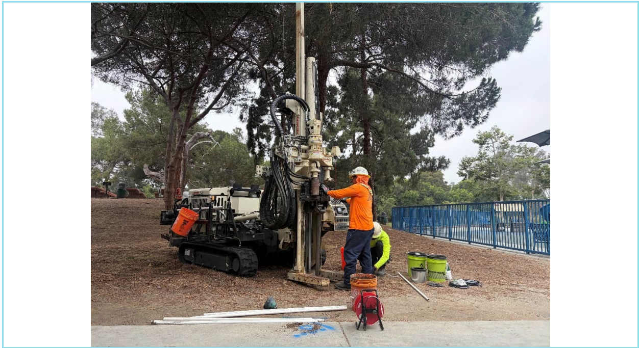
Photo 3: Drilling at SGP-3 and SGP-4.
