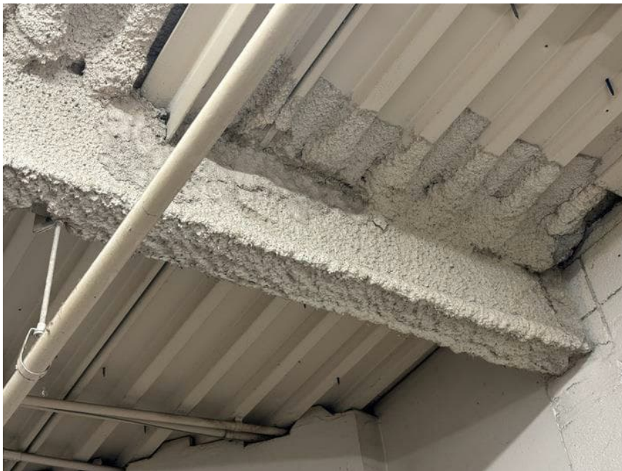
HA 15 - Spray-Applied Fireproofing
