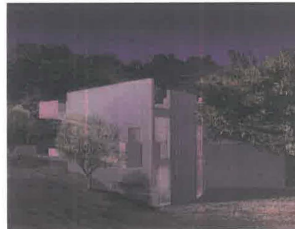
B3 - WEST AND EAST ELEVATIONS LOOKING NORTH FROM CLIFF RESIDENCE SOUTH
