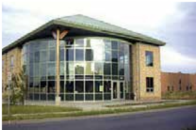
Example of industrial façade treatments
