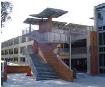
Solar panels on top of parking structure
