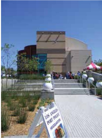
Los Angeles Port Police Headquarters
