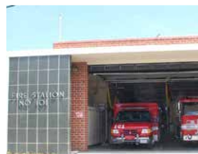
Fire Station 101 on W. 25th Street
