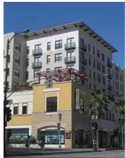
Example of a mixed-use development
