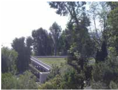
Green roof of a parking structure
