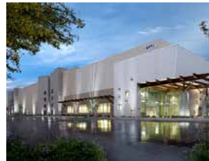
Prominent entrances to an industrial building
